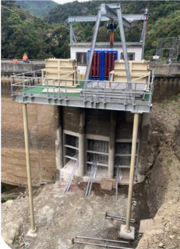
Upgrading intake structure for 4 station
