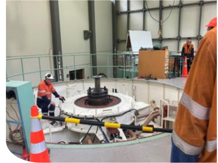
Maintenance works at 2a station
