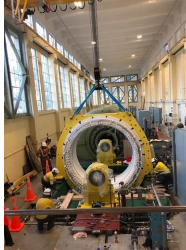
New G3 being installed
