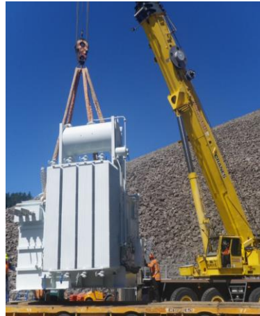
Transformer lifted onto trailer for short journey to switchyard
