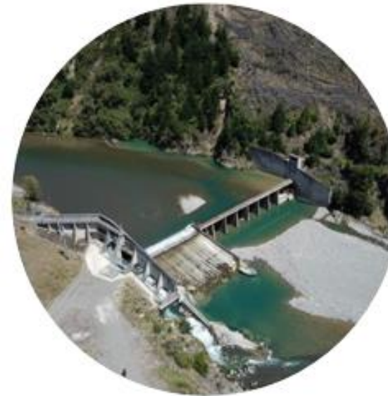
Aerial view of existing intake
