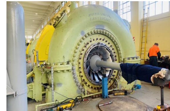
Coleridge G2 new runner and shaft install
