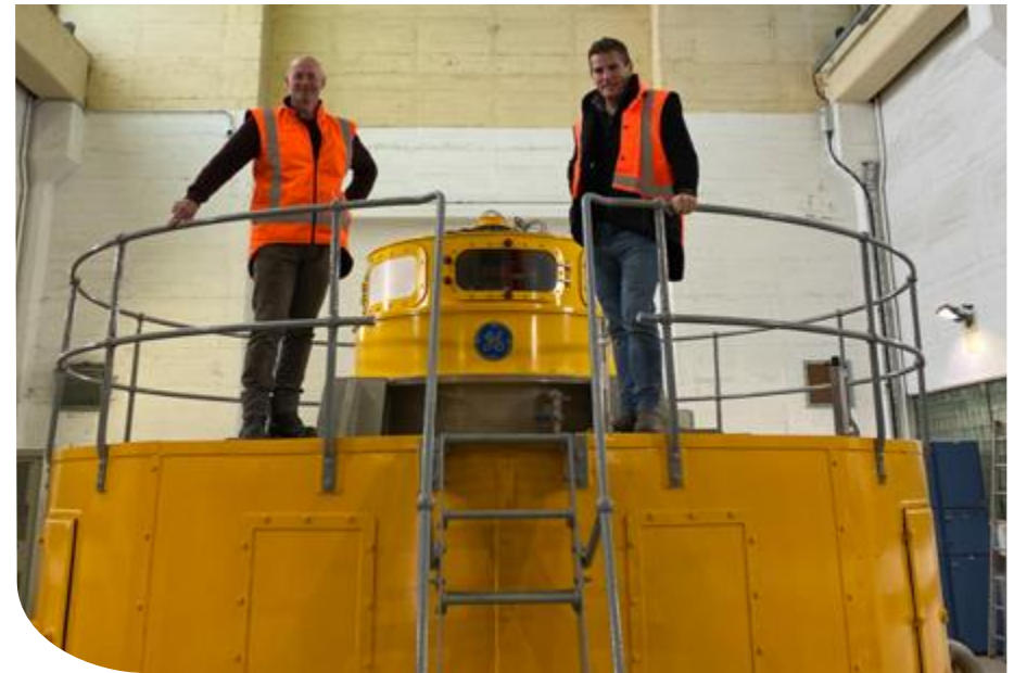
Stephen Fraser (GM Generation) and David Prentice (CE) at the newly commissioned Waipori 4 station generator
