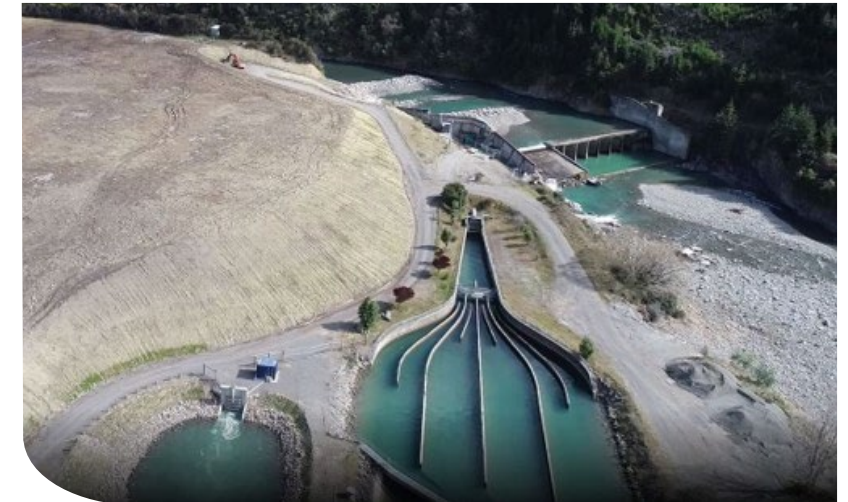
New Branch infiltration gallery with discharge into the Argyle Canal
