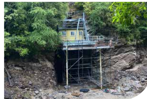
Waipori station maintenance underway
