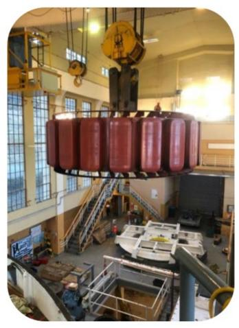
Highbank rotor being lifted into the stator
