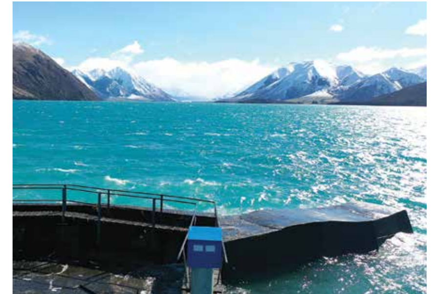
Lake Coleridge intake.
