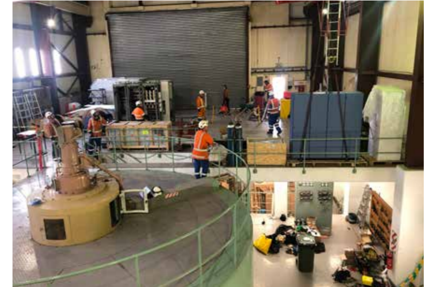
Some of our Waipori team at work in the power scheme.
