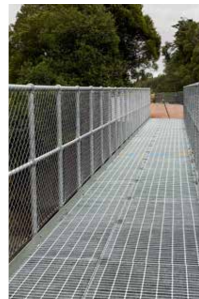
Renovated steel walkway, used by West Coast Wilderness Trail.
