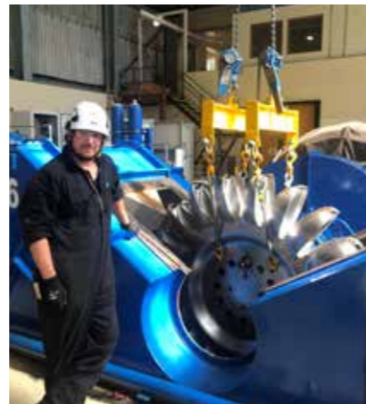
New Cobb runner installed.
