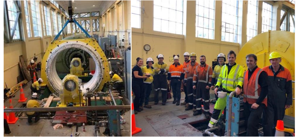
New G3 being installed
