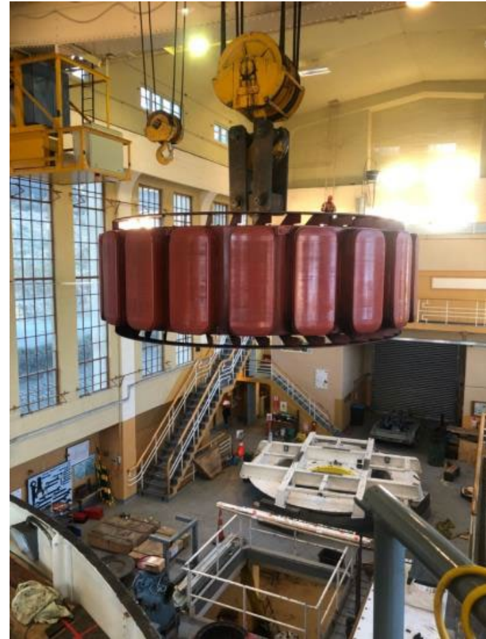
Bearing Housing put in place ready for alignment
